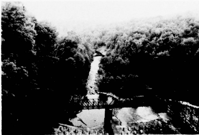
L. View of Downstream Channel from Spillway
